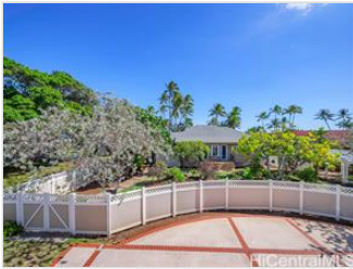
Makai view of the Main Home built in 1942 w/ 2,742 sf & updated w/ a remodeled kitchen, new paint.
