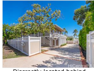
Discreetly located behind aesthetically pleasing privacy walls.
